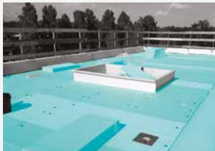
Achieving proper roof slope with FIBRANxps INCLINE boards and installation of FIBRANxps boards on a non-ballasted roof.
