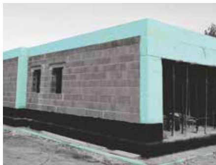
Insulation of thermal bridges on tie beams with FIBRANxps ETICS.
