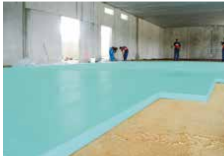
Thermal insulation of warehouse floors using FIBRANxps 300-L.
