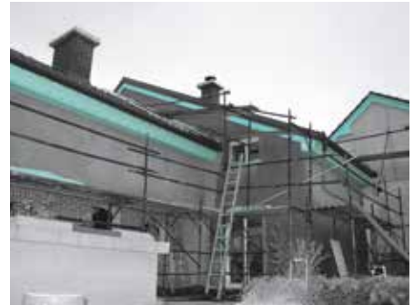
Roof overhangs covered with FIBRANxps ETICS. Thickness depends on construction span.
