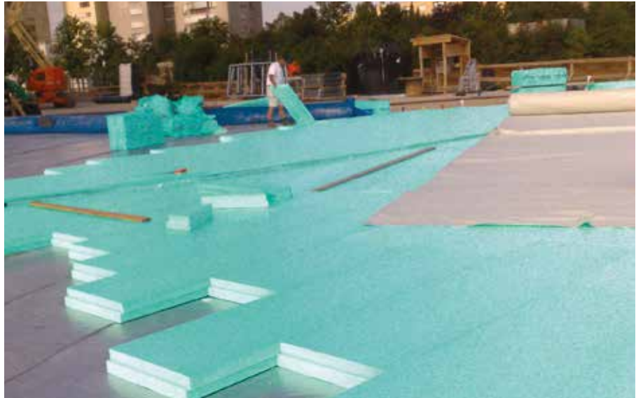
Full utilization of your roof - lining the inverted flat roof with FIBRANxps 300-L thermal insulation.
