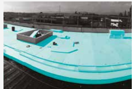
Achieving proper roof slope with FIBRANxps INCLINE boards and installation of FIBRANxps boards on a non-ballasted roof.
