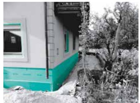
Resolving thermal bridges on window and door jambs and thermal insulation of façade plinths with FIBRANxps ETICS.
