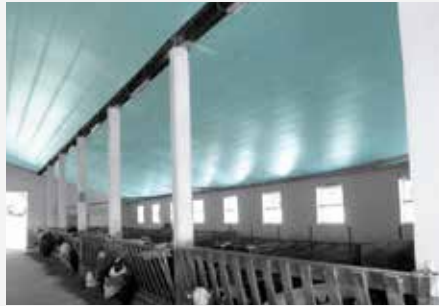
Visible thermal insulation FIBRANxps MAESTRO protects stables and agricultural buildings from overheating in the summer and cooling in the winter.
