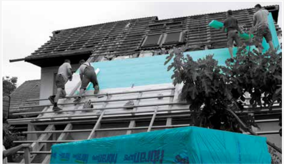
Energy-efficient system solution for the renovation of roofs over loft conversions in combination with a reflective roofing underlay FIBRANvent SILVER and thermal insulation FIBRANxps MAESTRO .
