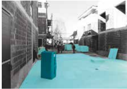
Incline solution and thermal protection of loaded platforms of residence buildings with basements with FIBRANxps 500-L and INCLINE boards.
