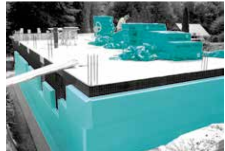
Solid, almost non-absorbent FIBRANxps 300-L insulation is a mechanical waterproofing membrane protection and permanent thermal protection of below grade parts of the building even in high ground water.
