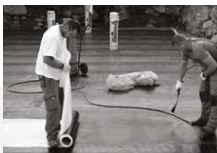
In the presence of ground water, the waterproofing membrane is laid in two layers: one-sided self-adhesive waterproofing FIBRANhydro T-3 sk and two-sided self-adhesive waterproofing FIBRANhydro SEISMIC T-1,8 sk/sk.
